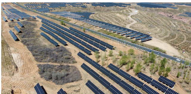
Photovoltaic panels at the Boortai Coal Mine, Inner Mongolia region, China.
